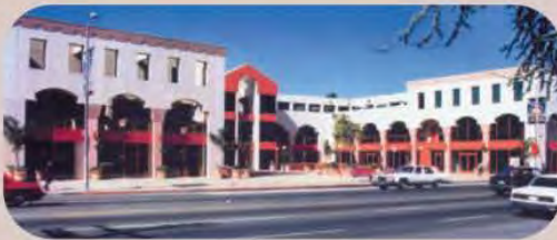
The Encino Spectrum Home of the Motion Picture Association of America Ventura Blvd. at Firmament, Encino CA Mixed-use project with 3 level underground parking 1995
