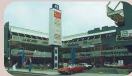
2130 S. Sawtelle Ave., West Los Angeles CA AIA award-winning retail office complex in West Los Angeles 1988
